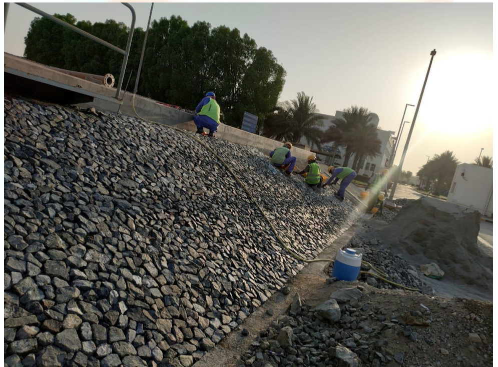
Laying of Rip-Rap Stone at NMDC Base, Mussafah
