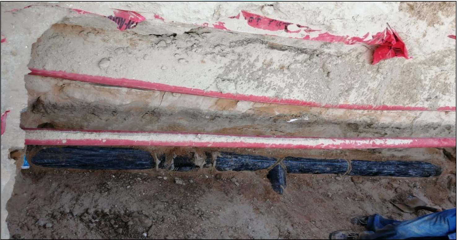
DI and HDPE pipeline work
