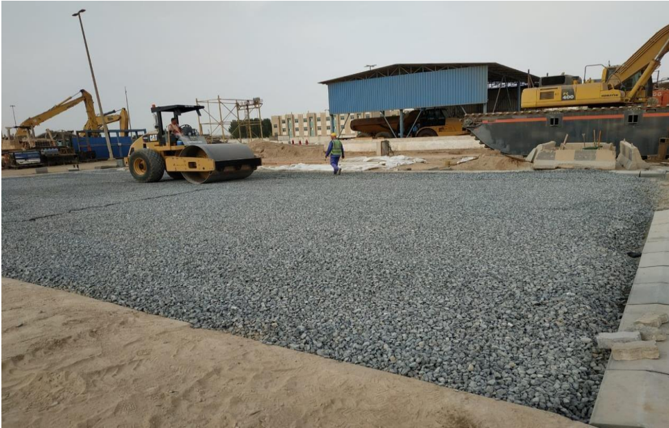
Laying of Crushed Aggregate at NMDC Base, Mussafah
